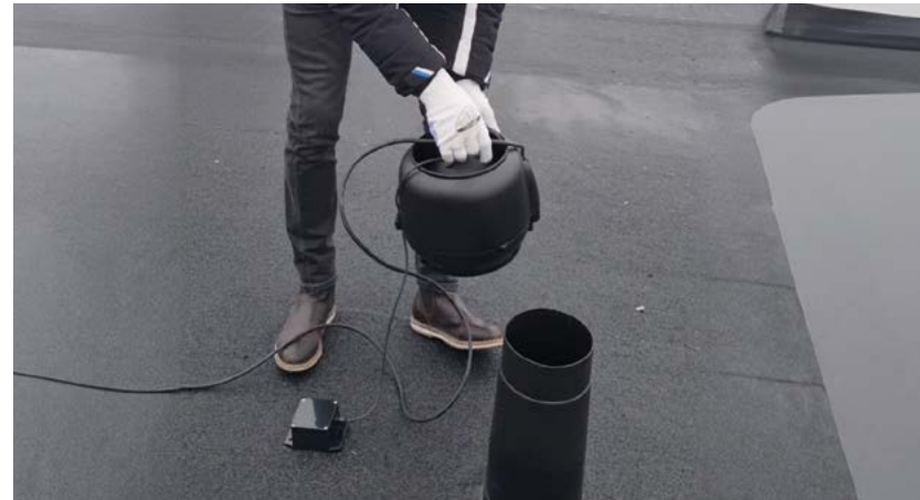
The VILPE Sense ECo roof fan installed retroactively on an VILPE Alipai underpressure vent.
