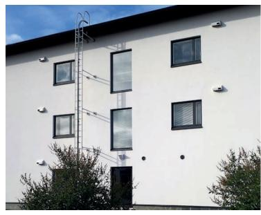
The exhaust air section of the IO Wall Element should be covered if the ventilation unit is switched off or not in use for a longer time period (for instance, in connection with the installation).
