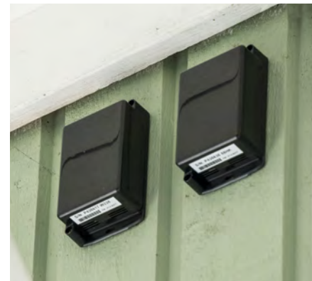
To the left: The VILPE Sense outdoor sensors on the outside wall. The housing company has two VILPE Sense systems and, therefore, two outdoor air sensors. To the right: The VILPE Sense indoor sensor in the crawl space.
