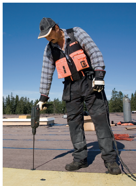
Installation of a felt roof using VILPE fasteners.
