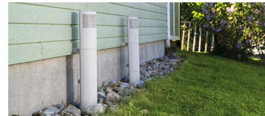
The crawl space has VILPE Ross ventilation poles which bring replacement air into the crawl space.
