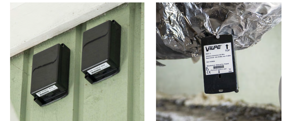
To the right: The VILPE Sense outside sensors on the outside wall. The housing company has two VILPE Sense systems and, therefore, two outdoor air sensors. To the left: The VILPE Sense indoor sensor in the crawl space.
