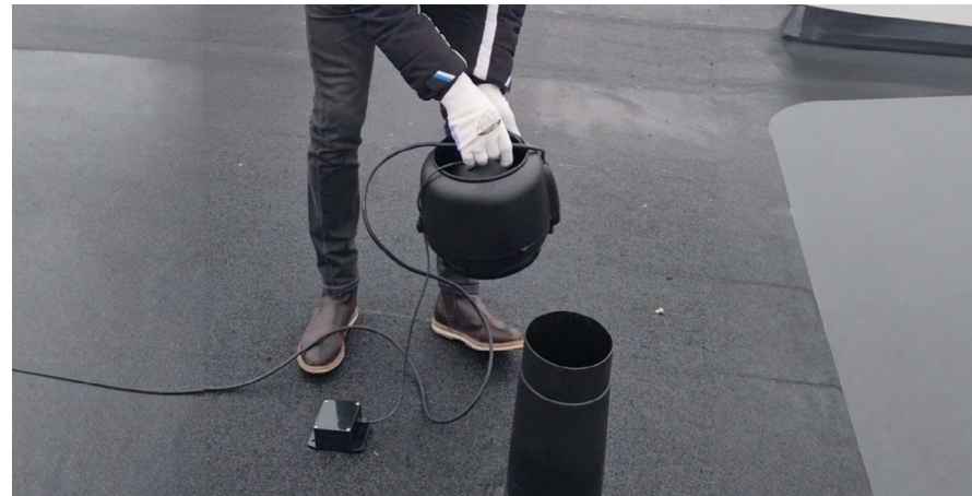
The VILPE Sense ECo roof fan installed retroactively on an VILPE Alipai underpressure vent.
