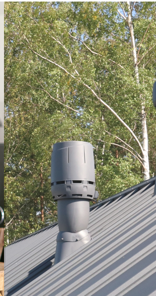
Kitchen cooker hood and a fan on the roof – silent kitchen
