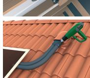
4. Shrink the shrinking tube with warm-air heater. Cable sealing is not shrunk or heated.
